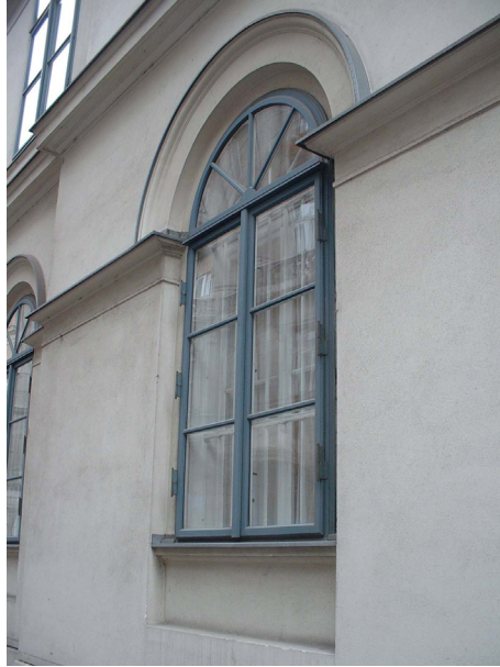
Fig. 6. The window manufactured according to Fig. 5 drawings in 2004 (age: 7 years)
