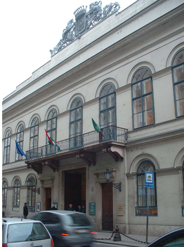
Fig. 1. The Károlyi Palace in Budapest – building envelope refurbished in 1996-97 – design and supervision by authors
