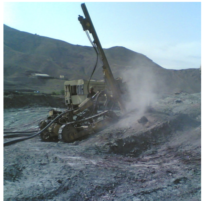
Fig. 7 Drill wagon machine in the studied mine
