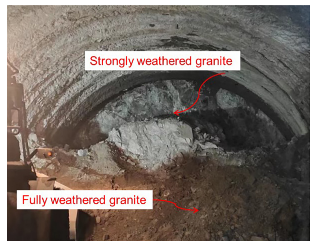
Fig. 1 The field geology of the tunnel excavation face
