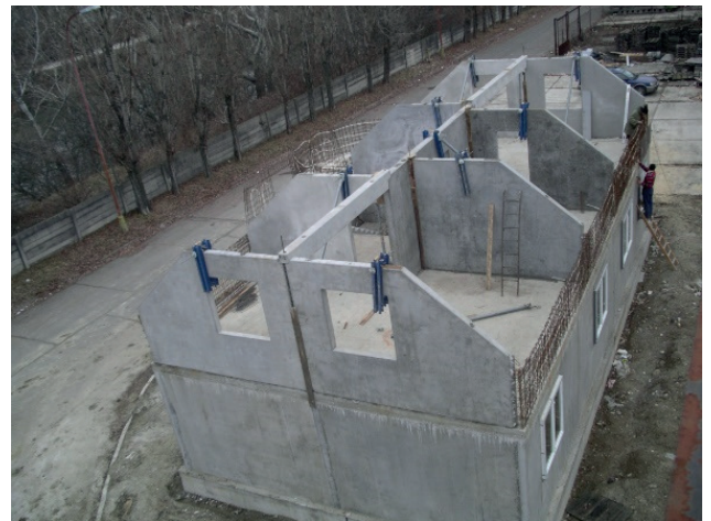
Fig. 6 View of the attic assembly (Photo archive: Kalús, D.) [2]
