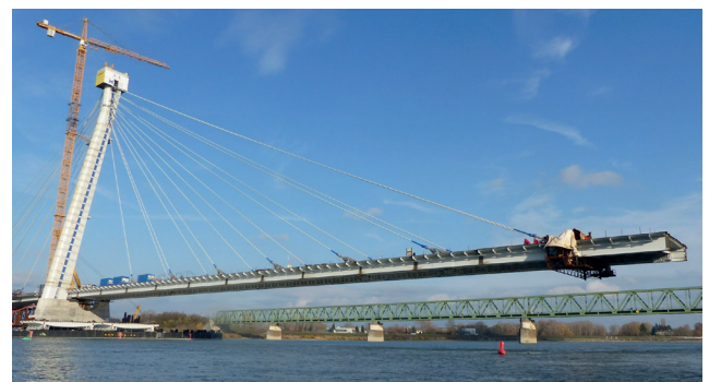
Fig. 2 Free cantilever of the bridge (courtesy of Pont-TERV Ltd.)
