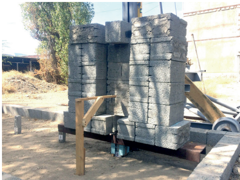
Fig. 3 Pile driving and static loading tests
