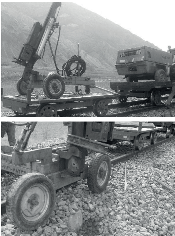
Fig. 5 Installing the lateral supports in ballasted track
