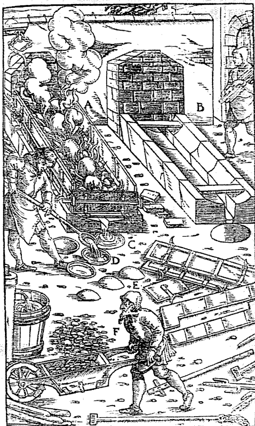
Fig. 2. Liquation furnace (Agricola: De re metallica 1556)
